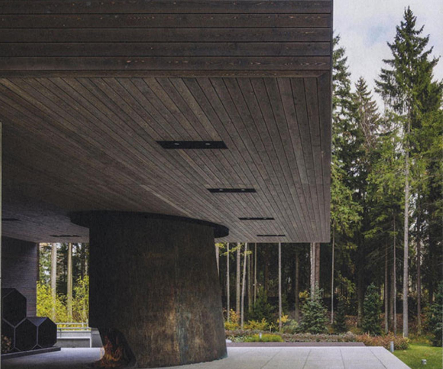
Detail of the custom cast bronze fireplace, the central feature of the portico on the ground floor, custom-made by an Italian art foundry. The parts were assembled and finished at the site.
