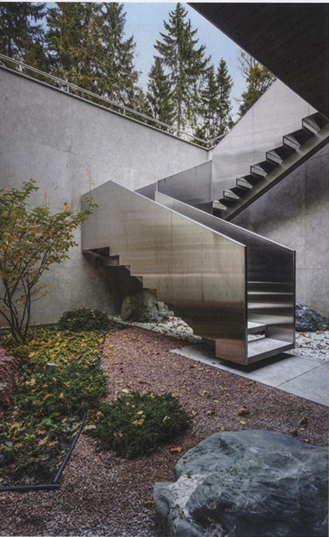
View of the external staircase in stainless steel and stone, connecting the garden to the entertainment zone complete with wine cellar, cinema and spa in the basement. A small Zen garden is located in the open area facing the cellar, conceived to bring air and light to the underground spaces.
